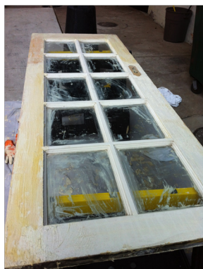
One of the two French doors during the stripping process
